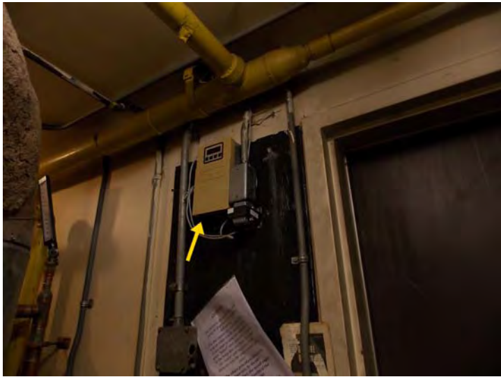
The boiler plant controller (arrow) uses outside air and return water temperature inputs to govern the boiler plant.
