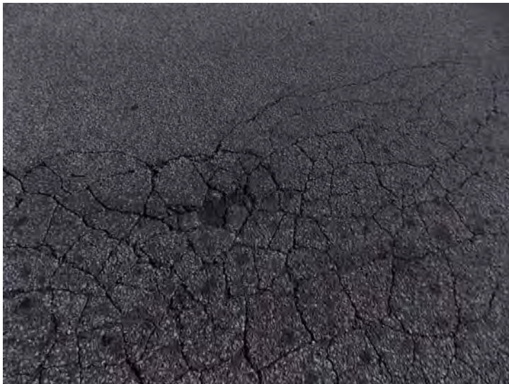
A close-up of a damaged section of asphalt paving.
