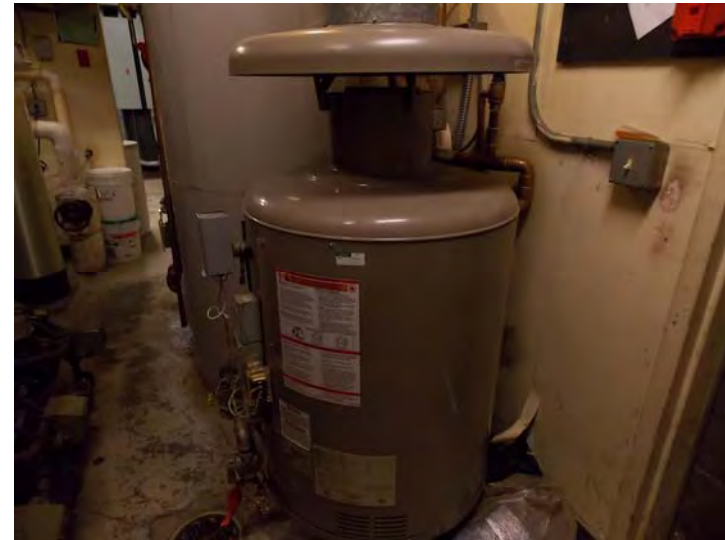
This is the natural gas-fired DHW boiler.
