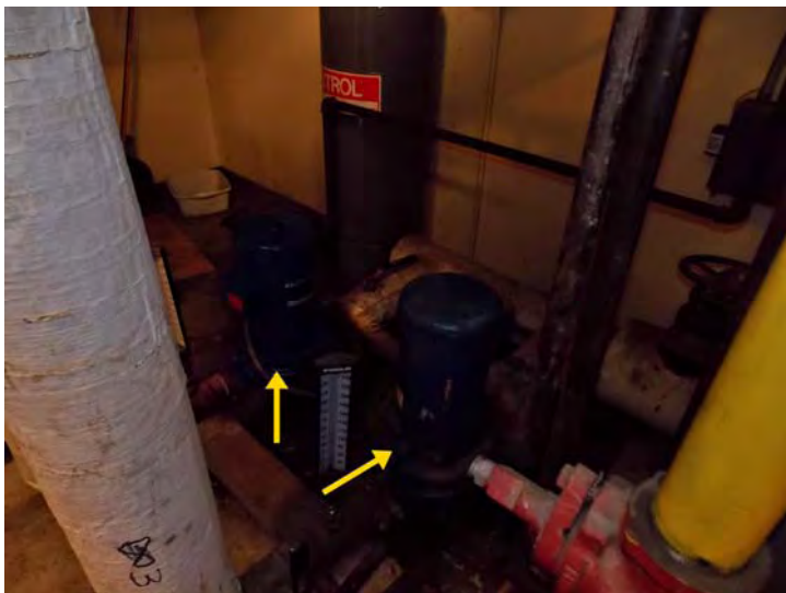
These are the two hydronic circulating pumps.
