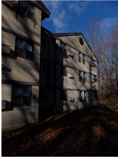
The building has three levels and is clad with synthetic stucco (EIFS).
