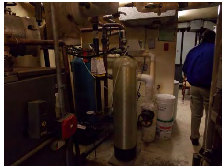
The mechanical room also includes a domestic water filtration system.
