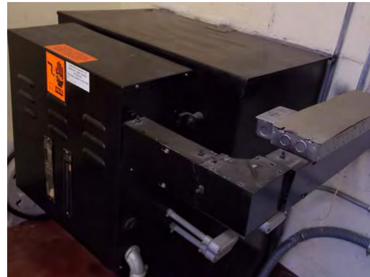
This is the elevator's hydraulic pump station.
