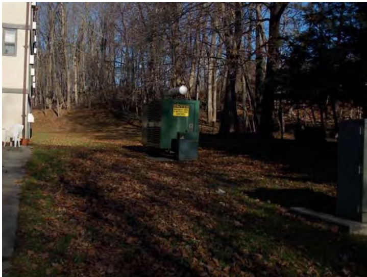
Emergency power is provided by this diesel powered generator.
